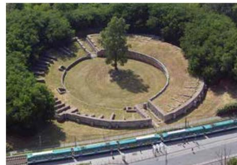
Built in the mid 2nd century, close to the north city wall. The ground plan is almost circular, the arena being 53.5 m x 45.5 m. The grandstand for 6-7000 people was around 15 metres wide. The outer curtain wall was reinforced with buttresses. The ring was surrounded by a stone wall around 3 metres high. On the stone blocks which served as seats, the names of the onetime owners have survived in places, including the names of women.
